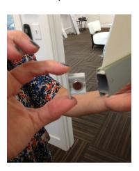
7. Roll down blind to make sure magnets in hembar and in door line up and locks into place.
